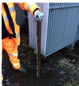
An operative was accessing Purley Substation compound when he walked slightly off path, stepping into what he thought was a puddle. However, it turned out to be a manhole with a missing cover, approximately one meter deep filled with water. The operative suffered a scrape to his shin, but the incident had the potential to be much more serious.
