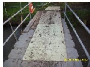
In a separate incident, an operative slipped on the central walkway at the River Avon site and fell on his side. He suffered strained abdominal muscles. The lighting over the bridge was fixed just above head height which affected visibility along the viaduct in the dark and wet conditions.
