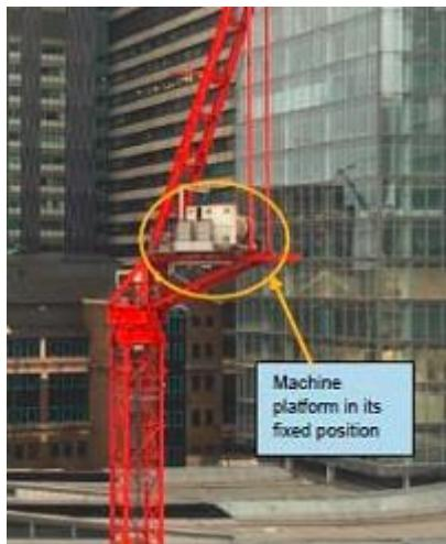
Whilst a mobile crane was being used to dismantle a tower crane at London Bridge Station, a load (hoist drum) became unstable and inverted. As a result, objects including two 2.5m scaffold tubes fell from the load. The scaffold tubes struck the newly installed canopy of Platform 10 and a train carriage berthed at Platform 11. Fortunately, no one was hurt, but it could have been much more serious. [Click on the image for full bulletin.](#)
