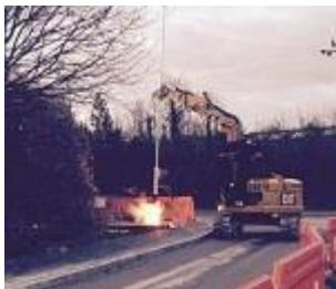
You can find the safety bulletin from the [Basingstoke incident here](#). You may want to use this as a basis for a tool box talk and a reminder on what you need to consider when planning works around overhead lines, and the potential serious consequences of not having a robust plan in place.
