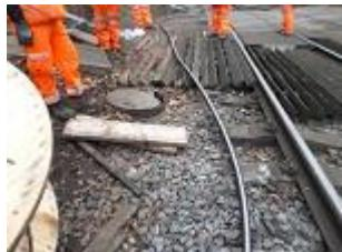
During works at Englemere Level Crossing, an operative stepped on a plastic turning chamber that was covered in leaves. His foot went through the cover causing bruising to the foot and he was taken to hospital for X-rays.
