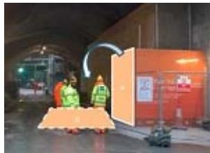
During Thameslink works at London Bridge, a vehicle access gate detached from the gate post and fell to the ground. The gate is four metres wide by three metres high and weighs approximately 400kg.
