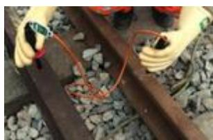
Under the Southern Shield charter, it is also a requirement that everyone in the working group observes the COSS testing the conductor rail and signs the SSOW pack to confirm they have witnessed the test.
