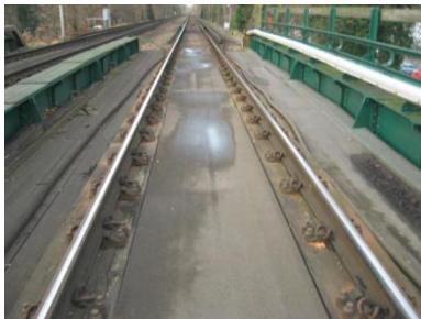
A maintenance operative was carrying out inspections on a timber bridge when he decided to crossover the wet walk boards, rather than walk around the ballast. As he was walking across to the down road, he slipped on the timber and hit his left hip and knee on the running rail.
