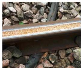
The scrap rail had been placed in the 6ft by Works Delivery during installation of new rail; however, an engineering train prevented the team from removing the scrap rail during later shifts. A decision was made to leave the scrap rail in place until a suitable possession was identified.
