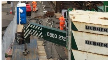
**Background:** A 750 tonne mobile land crane was employed to replace Aldershot High Street Bridge within a 52 hour possession. Crane mats were installed to spread the load from the outriggers so that the pavement, carriageway and buried services were protected.
