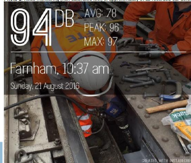
Photo 2: noise monitoring (non calibrated tool) of approximately 97db recorded-ear defenders worn
