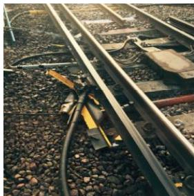
Following works in a line blockage at Ascot Station, a train struck two conductor rail shrouds on the down main line. The line blockage was set up by a Protection Controller (PC) with a number of COSS's undertaking a range of works on and around the station platforms. Conductor rail shrouds were deployed for each of these operations.
