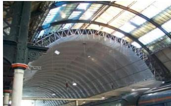
An alternative scenario to the one mentioned above would be the designer specifying that the scaffold is suspended from the existing bridge structure and leaving the detailed calculations to the scaffold contractor. In this scenario, the scaffolding contractor may not be aware that the bridge itself will need to be assessed to ensure it has sufficient spare capacity to support the scaffold.
