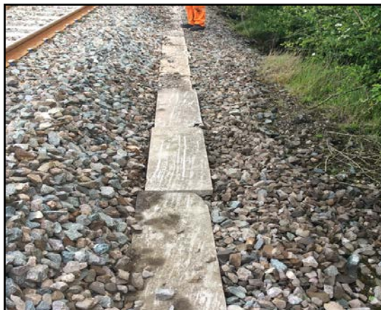
BML3 163m 15ch - Gap in the Troughing route
