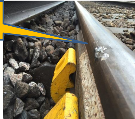
Damage to Rail
