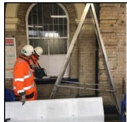
On the Reading 10 Car project electricians were seen working from a step ladder without an appropriate exclusion zone. Commuters were using the bench below whilst the works were taking place. The works were stopped and a safety conversation was held with the electricians to discuss working practices.
