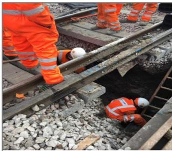
As part of signalling and track works, an under track crossing (UTX) was required to be installed at New Cross station. An excavation was needed which passed under three tracks from the cess to the station platform.
