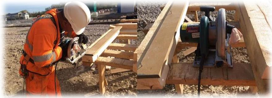
A construction manager stopped an operative working on site after seeing him using a circular saw, which had a piece of cloth jammed into the dust extraction port. This cloth could have jammed the saw; making the saw jump and potentially injuring the operative.
