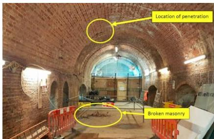
The shoulder of an arch at the London Bridge Station redevelopment project was breached. This was as a result of excavating overburden for the formation of a pin for a structural ground beam. The excavator operator became aware of the penetration, stopped work and reported the incident to his supervisor.
