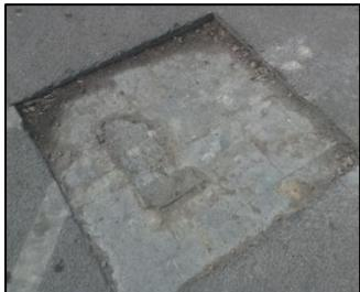
A Close Call was raised after 100 millimetre holes were left in the site compound at Ascot Station car park. The holes were left as a result of the concrete supports to site office being removed. This caused a trip hazard, so the site manager instructed staff to place chapter 8 barriers around the holes and fill it with type 1 to eliminate any further risk.
