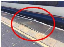
A Close Call was raised after a member of the team in IP Wessex spotted that two of the coper stones were causing a trip hazard at Havant Station. The stones buckled and were raised above the normal platform level by around 30 millimetres. This was causing a tripping hazard to the public at the platform edge, and also potentially a risk of a person being hit by a train.
