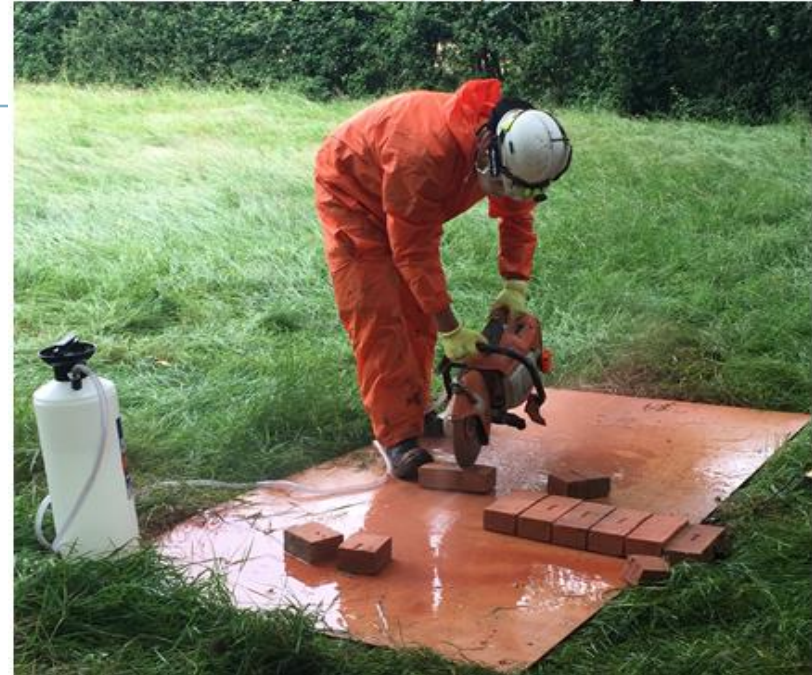
Photo 2: Wet brick cutting with full PPE in place including a coverall
