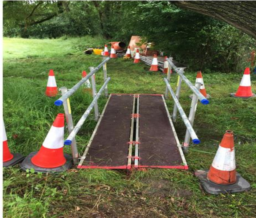
Photo 1: Good practice: Staging boards marked and used for safe crossing
