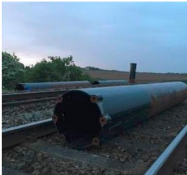
So the work group installed the pile to a safe depth and travelled back to the access point approximately 20 minutes away. No-one on-site remembered to collect the pile which had been set down in the four foot.
