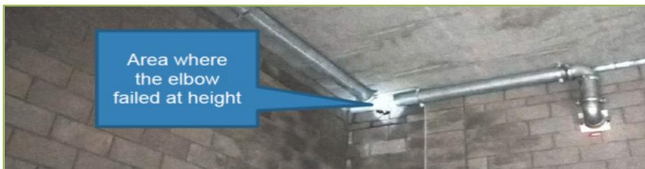
The failure occurred at a 90 degree elbow which is approximately five metres from ground level. No one was injured but the event is being treated as significant due to the potential for injury to persons on site had the failure occurred at another point in the system.
