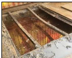
In this instance had a Close Call not been raised a vehicle could slide into the pit or the dislodged plate could have moved further and hit someone while a vehicle was travelling over it.
