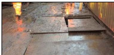
A Close Call was raised after a fully laden HIAB lorry drove over metal road surface plates and displaced them exposing a 1.5 metre deep pit of sludge and waste water. The lorry was being driven through a skip company's yard which led to an access point to Network Rail land. To get there the lorry had to cross over an area covered with steel road plates, the area was dirtied with mud and waste oils.
