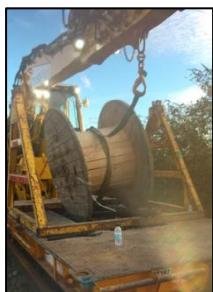
A team was lifting and removing an empty cable drum. It was located on an A frame attachment and mounted on a rail trailer. The drum was being lifted using a strop and the weight taken from the spindle bar. As the drum was being lifted it slide through the hole of the drum, travelled through some bridge railings and fell to the ground in a public area. The spindle is believed to weigh around 40-50kg. This incident is currently under investigation.
