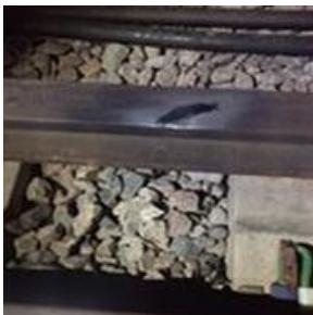
In another incident (photo), an earthing strap was dropped onto a Live Conductor Rail while a possession isolation was being taken by the Wessex Route team. This caused a flashover and the individual was taken to hospital to have an eyesight check.
