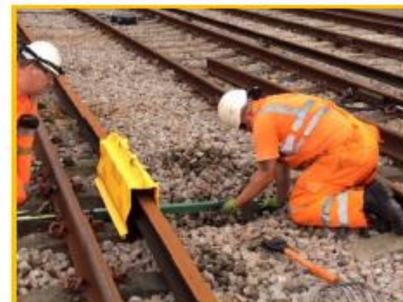
Figure 1. Fitting under the running rail and adjacent conductor rail.
