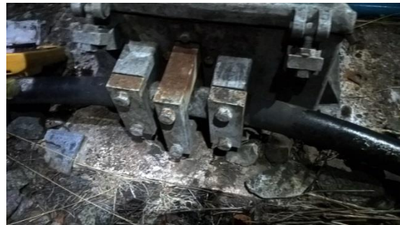
Figure 2. 750v dc cable clamps masking damage.
