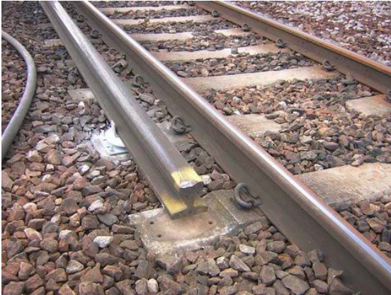
Ramp end with impact damage and bracket that hit passenger on the platform
