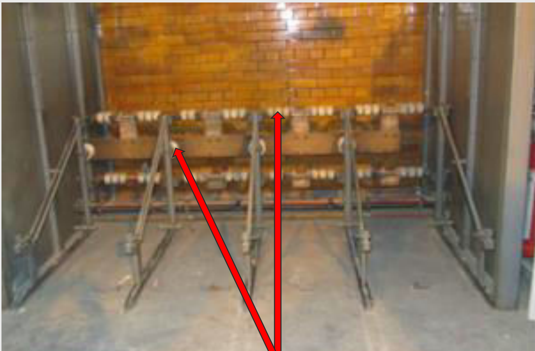
Packers / spacers (DC Busbars)
