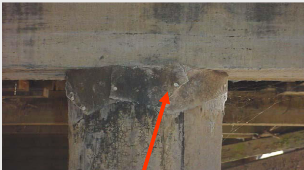
Roofing felt pile cap on timber bridge.
