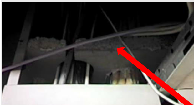
Insulating board with non-asbestos sprayed coating
