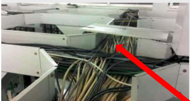
Debris within cable trays
