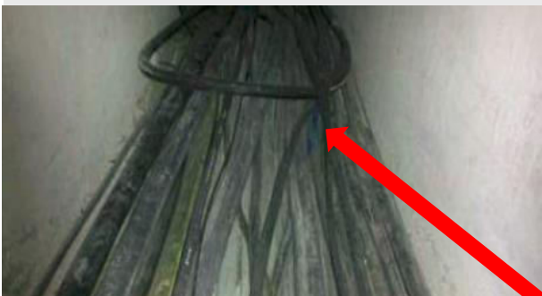
Debris within ducts
