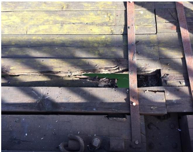
Until further notice the use of the timber walk way on this single line structure, is prohibited. The only pedestrian route across the structure is via the Girders
