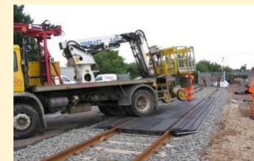
Fig 12 Temporary track access systems
