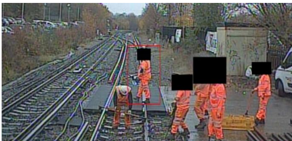
The PiC/COSS using the track gauge with his back to traffic, the Site lookout in the 4ft
