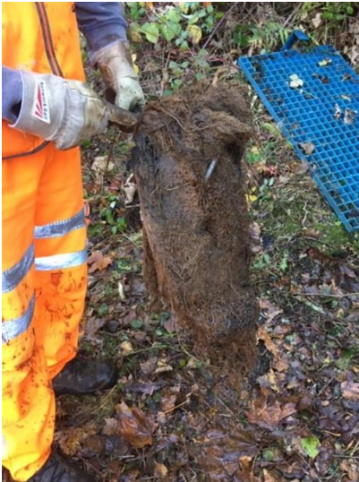
Roots removed using the 'Pigs Tail'
