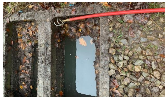
'Pigs Tail' fixed to drainage rods resting on a catch-pit
