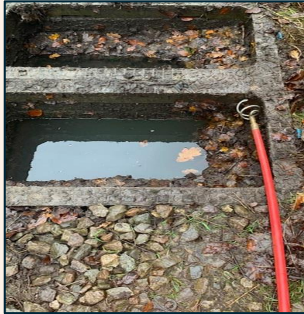
“Pigs Tail” attached to a drainage rod and roots removed using the attachment
