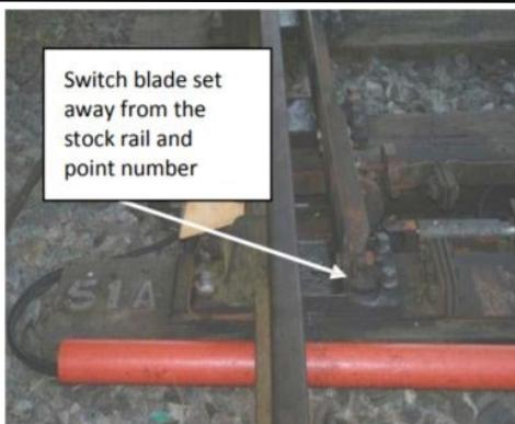
REVERSE POSITION (identified by the point identification plate closest to the OPEN end)
