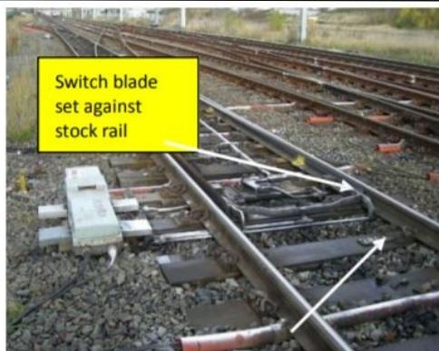
NORMAL POSITION (identified by the point identification plate closest to the CLOSED end)
