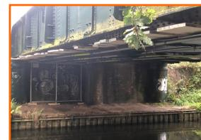
At this point, the black matting used to prevent debris falling into the canal, was concealing the fact that there were no boards in that section. He fell through the scaffold up to his waist before catching himself. The worker was bruised but sustained no significant injuries, however he was shaken by the incident.
