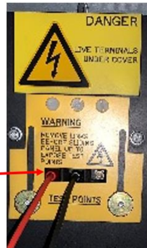
Test point with injection leads
